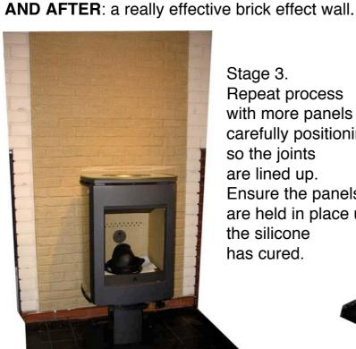
Stage 3. Repeat process with more panels carefully positioning so the joints are lined up. Ensure the panels are held in place until the silicone has cured.
