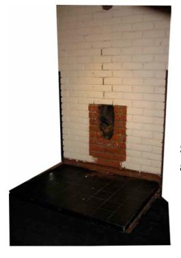
Stage 1. Apply half dozen blobs of high temperature silicone to the back of a Skamolex panel.
